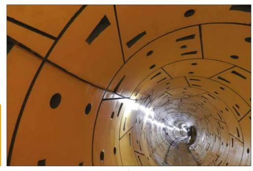
Technicore used Herrenknecht Combisegments on the West Tunnel Sewer Contract 2 in Mississauga, which requires no welding because gasket and liner are joined during the manufacturing process
